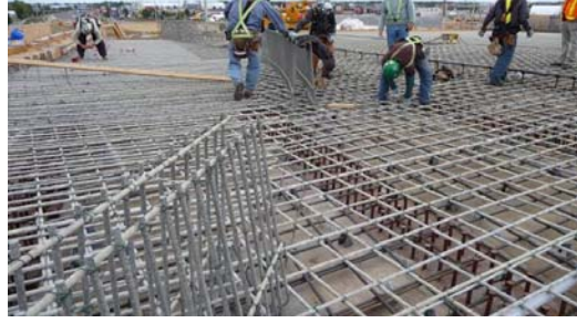
Figure 2: FRP decks/app slabs/ barriers, Skagit River – BC MOT (2009).
