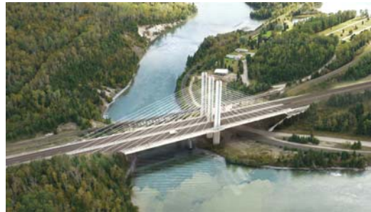
Figure 3: Cable stayed bridge, Nipigon River Bridge, ON (2015)
