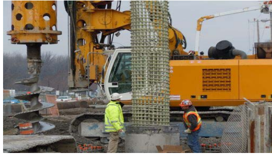
Figure 4: Handling and lifting the GFRP Soft-Eyes
