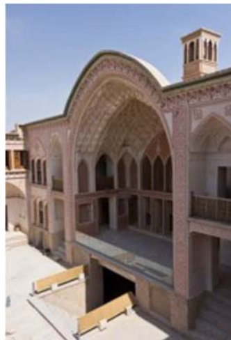
Figure 4 Iwan of a traditional building. Source: Ali, Alamoudi, Alajmi, Khayat and Aishraim, 2014.
