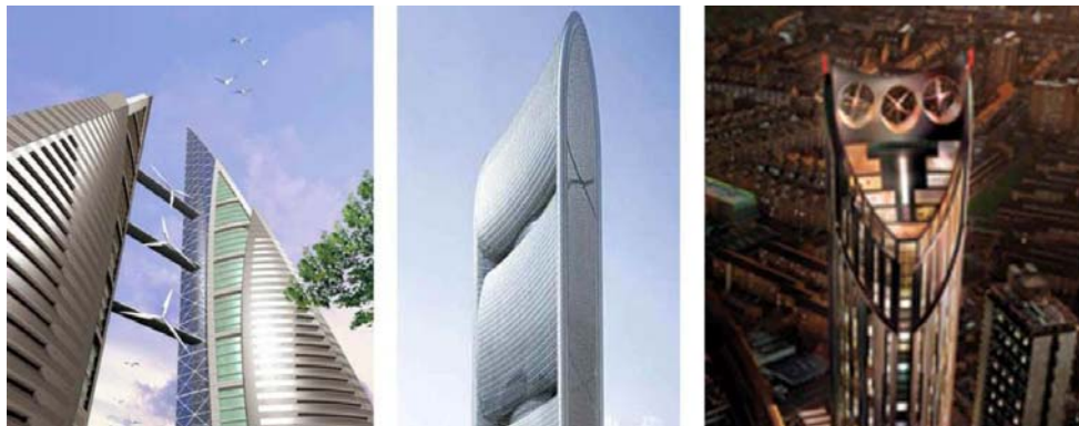
Figure 4 left to right: Bahrain World Trade Centre, Pearl River Tower in China, Strata SE1 project in London.
